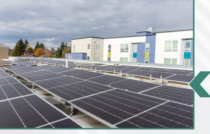
168 Solar Array providing 80.64KW power
